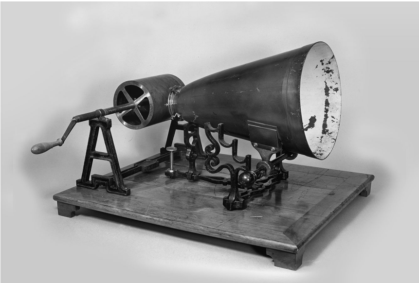
FIGURE 1.2 Phonautograph, patented in 1857 by Édouard-Léon Scott de Martinville, built by Rudolph Koenig, and purchased in 1866 by Joseph Henry, first secretary of the Smithsonian Institution.
